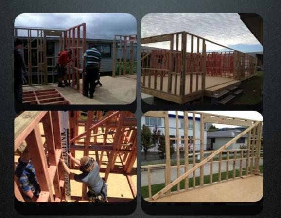
We Erected all the frames and tacked them in place. When all the frames we up we straightened all the joins and then braced it all straight using string lines.
