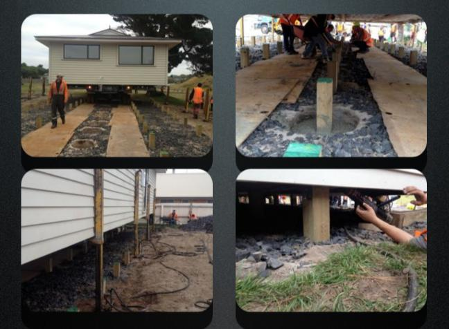
After getting the house to site, it is backed into place before being held up by jacks so the truck can get out. When the truck is gone the middle row of piles is concreted into pre-prepared holes. The house is then lowered onto the piles using hydraulic jacks .
